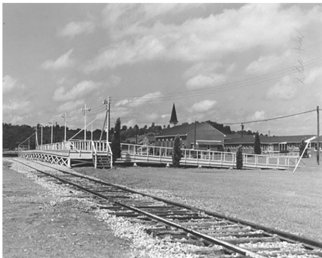
The Fletcher train platform and chapel.
